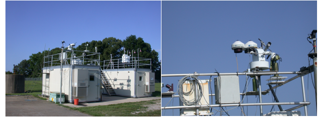
Calibration site at NASA Langley. Having a land location calibration site allows for greater opportunities to collect data on clear sky days. Compare to the multi-day lead time and logistics of a COVE-CLH trip, which requires a helicopter ride and predicting the weather a few days in advance. Pyranometers and pyrhemometers with their associated Campbell Scientific dataloggers are calibrated here as a set and then taken to COVE-CLH. This set is directly traceable to the World Radiation Group in Davos, Switzerland.
