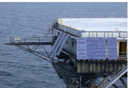
Upwelling instruments are at the end of the 8m catwalk on the west side of the structure.
