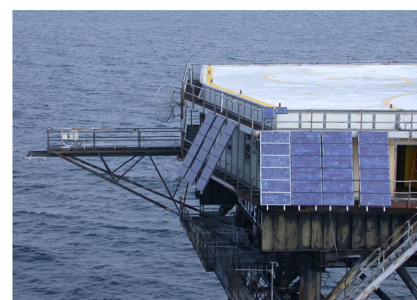
Upwelling instruments are at the end of the 8m catwalk on the west side of the structure.
